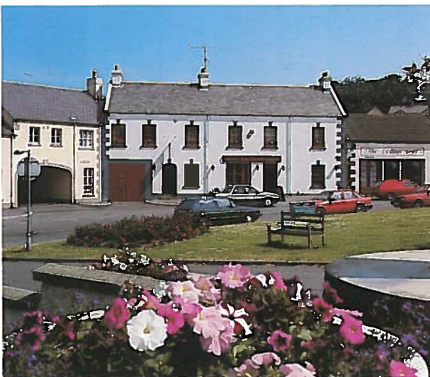
Developments should make a positive contribution to townscape - redevelopment and infill scheme, Strangford.
