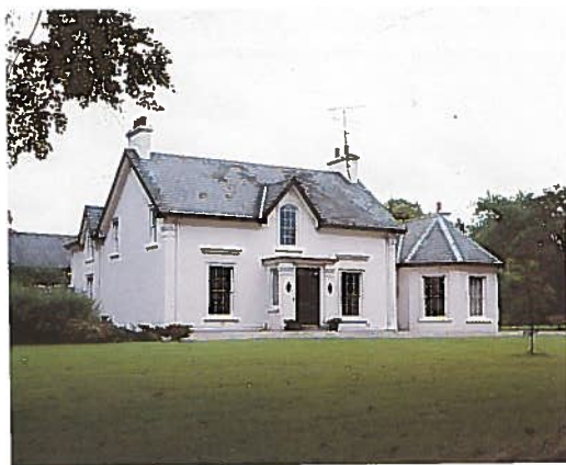
Replacement of dwelling destroyed by fire.
