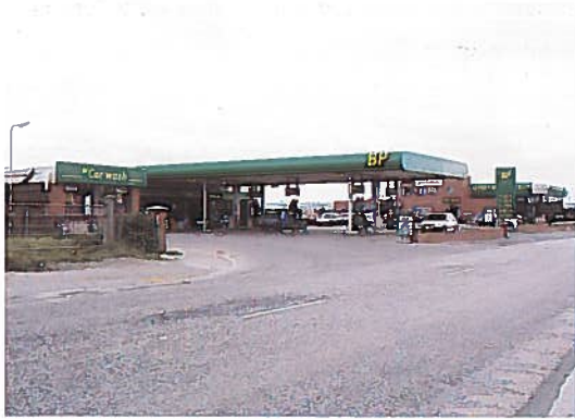
Roadside services for long distance travellers using the trunk roads network - Moira.
